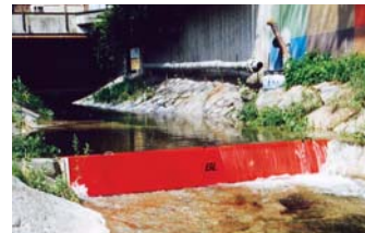
Retention barrier BL/BAP, manual system in the Superflex Line, permanently bolted in place
