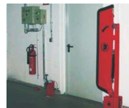
Retention barrier BL/BED-A, semiautomatic, damped automatic closing, manual resetting
