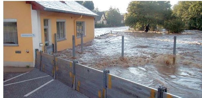
Flood protection wall BL/HSW-SB demountable Length: approx. 70M Retention height: 1m
