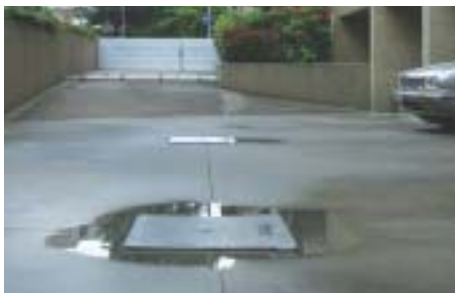
Stormwater inflow/overflow protection with Sealing Plate BL/FAP-P1, directly bolted.
