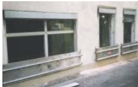
Window Seal BL/FAP-PR2 with frame and pressure rails.
